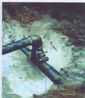
SPILL POINT [SP] 2 [3" BALL VALVE WITH CONNECTION]
